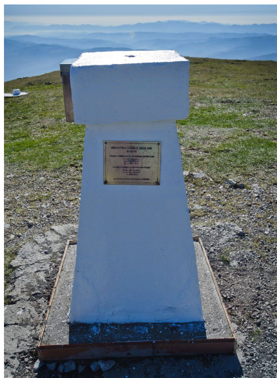
Figure 52: Topography of the first order point No 169 on Blegoš and a renovated pyramid that represents the point in space.
